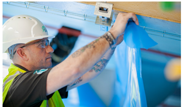
Asbestos Operative helping form an enclosure within one of the scaffolding zones.
