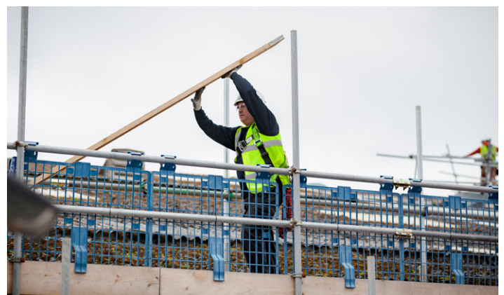
One of Shield's scaffolders forming an external gangway to aid the re-roofing project.
