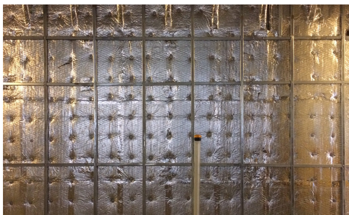
Completed A60 insulation Protocol applied to the newly installed steel bulkheads on two levels.
