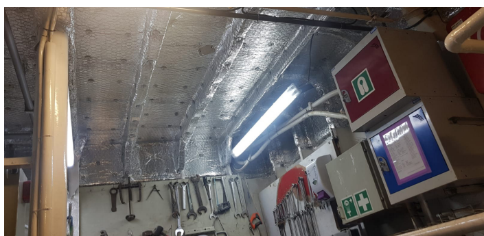
Completed A60 insulation Protocol applied to the newly installed steel bulkheads on two levels.
