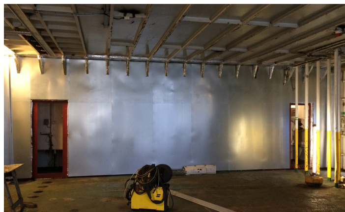
Cladding covering the insulation was installed as a separate application to prevent flammable fluid ingress and to offer mechanical protection against damage.
