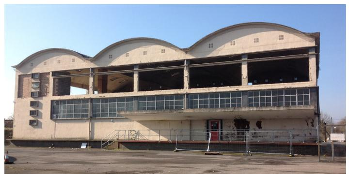
Former Bakery building after completion of works to roof and first floor areas. First floor perimeter walls along with full internal removal of all walls, wall coverings and floor screed was carried out as part of the asbestos remediation works.
