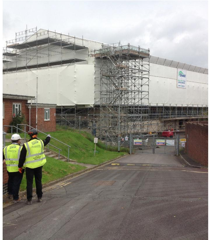
Example of challenges and works undertaken. Purpose built and designed fixed scaffolding erected over roof and first floor areas, to facilitate asbestos remediation works to these areas of the former Bakery Building within Bulford Barracks by SES.
