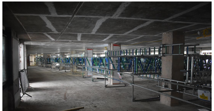
Internal view of truss-out assembly and anchoring assembly
