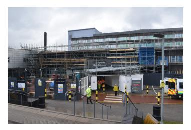
The contracted works involved fully stripping back to the original concrete 'shell' of the internal areas of work, which were undertaken under both semi and fully controlled conditions. All works were carried out in accordance with the Control of Asbestos Regulations 2012 (CAR2012), the Licenced Contractors Guide HSG247, and as a rolling phased programme
