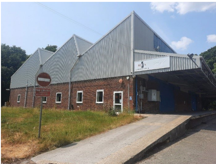
Units 6 & 7, Chalcroft Business Park
