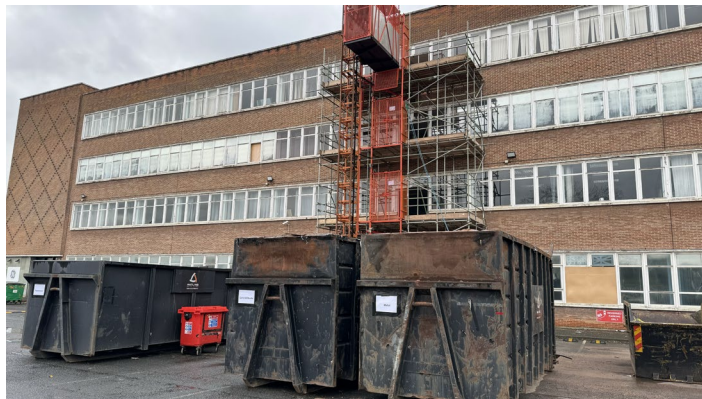
Hoist system helped to provide access to all floors
