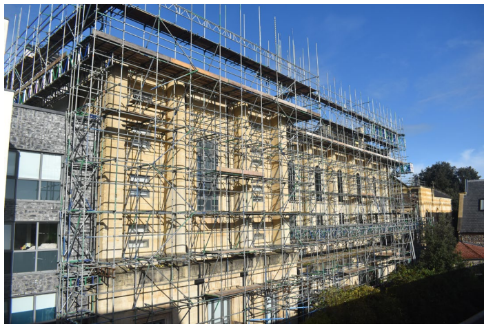
External scaffold structure ahead of HAKI roof system being constructed
