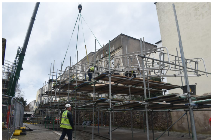
Jig with roof section in place prior to lift
