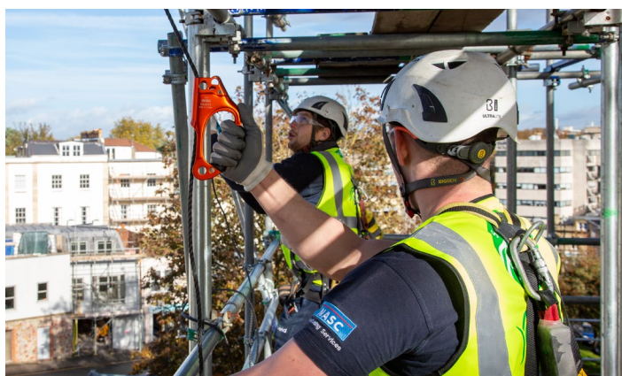
External scaffold structure ahead of HAKI roof system being constructed
