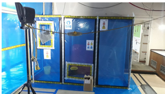
Example of airlock to live asbestos enclosure
