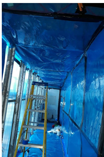
Left: Enclosure preparation to external mullions
